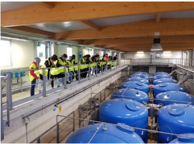
Figure 1. On-site visit of the Mancasale WWTP
